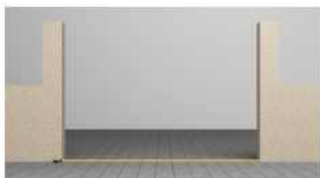
3 Mesurer en bas: Measure the distance between pillars at the bottom.
